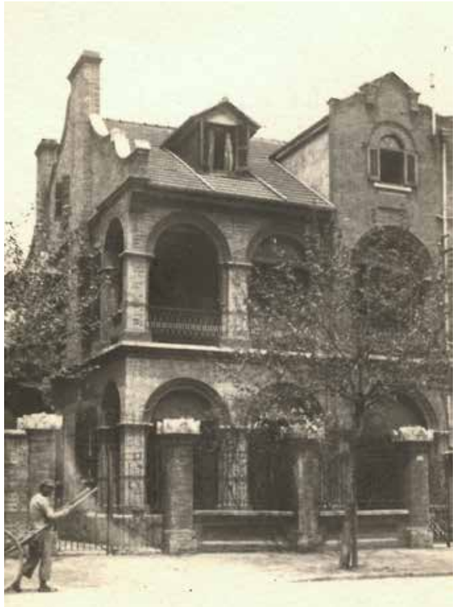
The Mess, Rue Bard.
