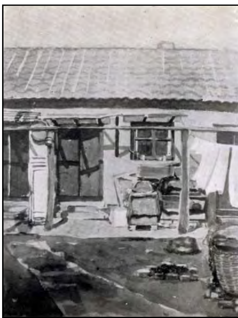
EXTERIOR OF AN " APARTMENT "
